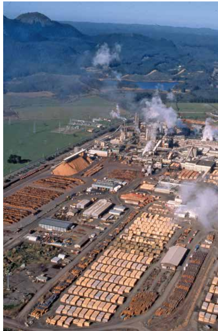
Kawerau wood processing site
