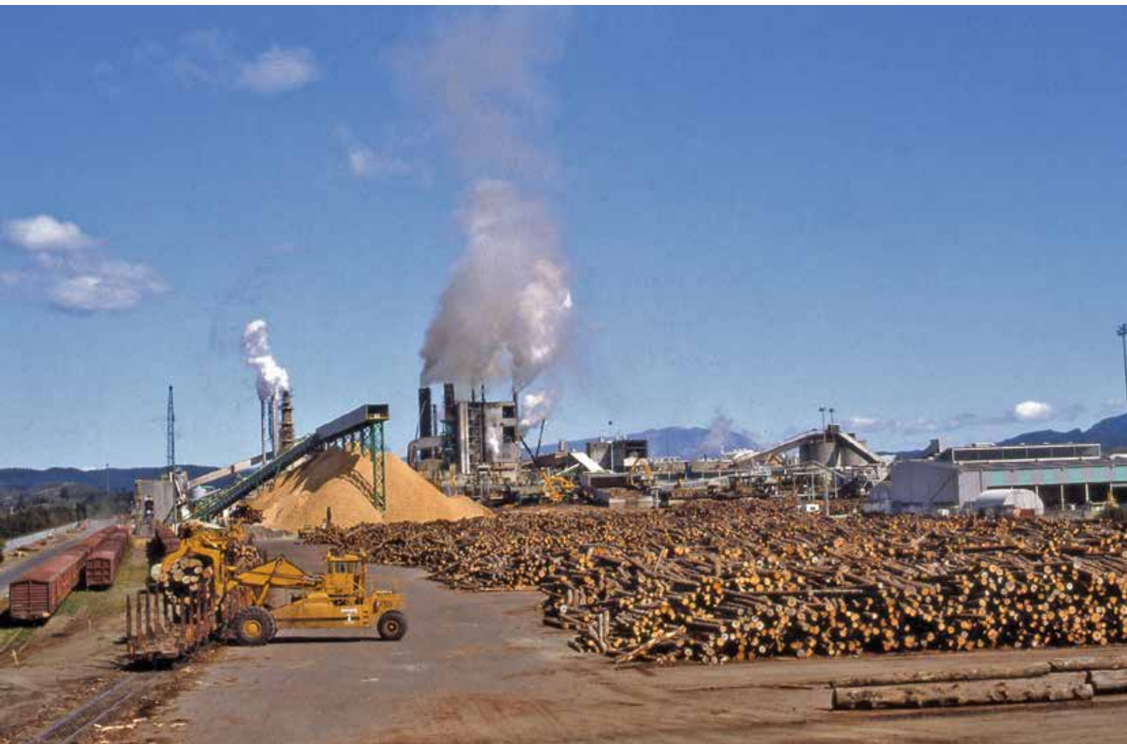
Kawerau pulp mill log yard
